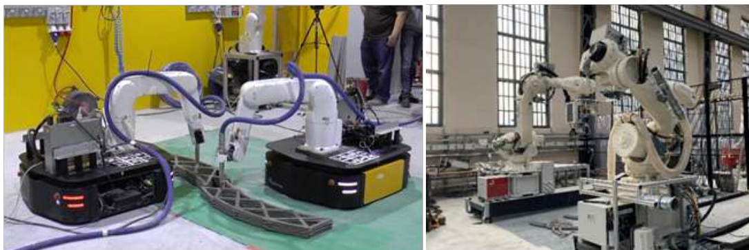
Figure 3: Mortar printing using cooperative mobile robots (Nanyang technological Univ. , Technical Univ. of Berlin)
